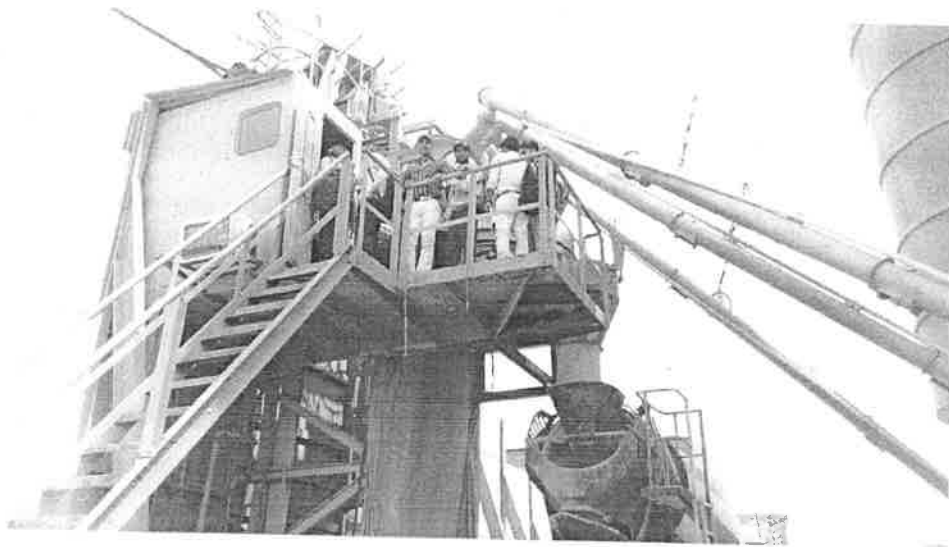
RMC loading in Transit Mixer
