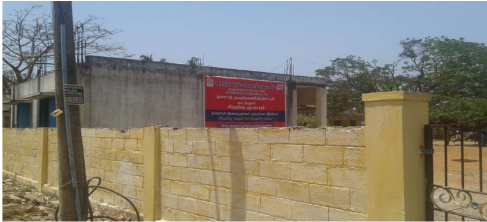
Wall Constructed by Our Nss Volunteers During the Special Camp at Paduvancherry Village.
