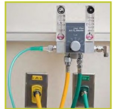
Figure 4.16. Flowmeter set to 10 L/min. Adjust blender to desired oxygen concentration.
