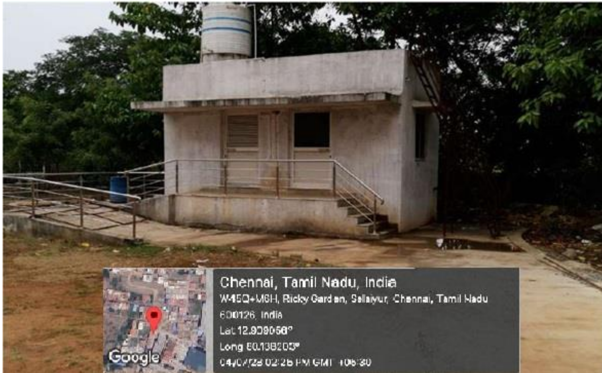
Waste Recycling Unit
